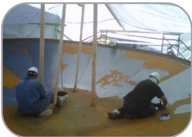
Mining project requiring metal resurfacing and rubber relining of 25' dia process tank.
