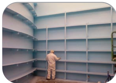
Food and Beverage project requiring existing coating removal and recoat with 100% solids novolac epoxy system.
