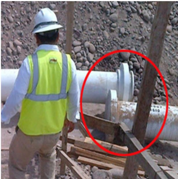
*Mechanical joints significantly complicate the construction process.*
