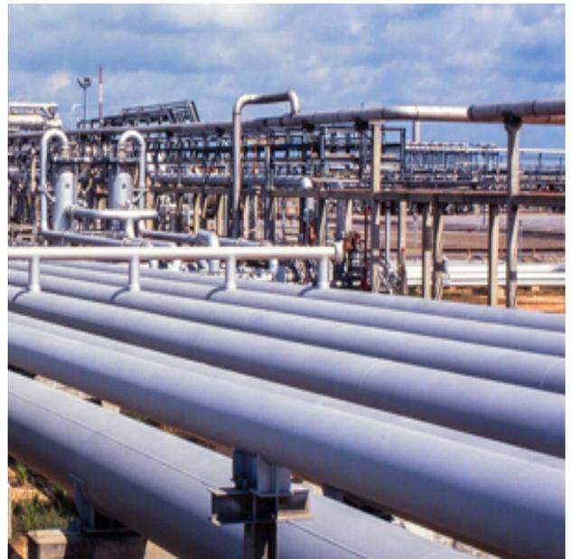
*Modifications are easy with welded joints, and the number of pipe supports can be reduced.*
