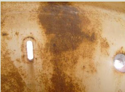
Severe steel corrosion in water filtration tank
