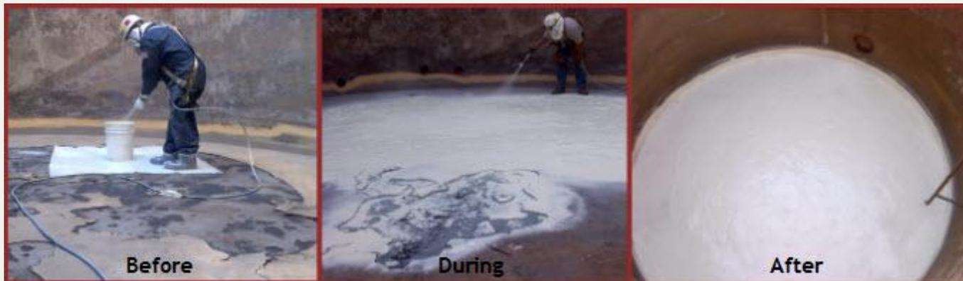
Holes were unexpectedly found on this tank floor only 48 hours before it needed to be filled. With no time for welding, Goodwest developed and implemented a single-coat solution that sealed the floor.
