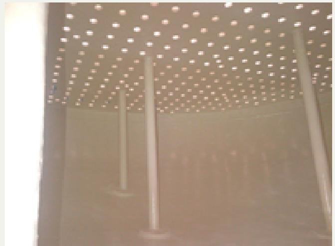
Goodwest engineered and installed an elastomeric polyurethane lining using the patented [ECOSYSTEM®](#) gas-expanded technology to create a 1/4” thick barrier between the saltwater and steel. This technology allows for thick-film buildup in a single coat on complex steel structures.
