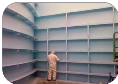
Food and Beverage project requiring existing coating removal and recoat with 100% solids novolac epoxy system.
